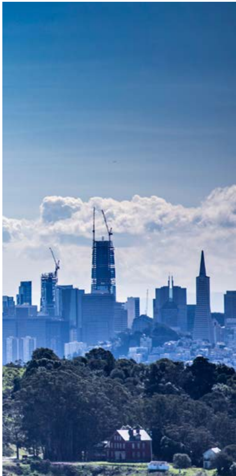
Construction in San Francisco. Credit: Karl Nielsen
